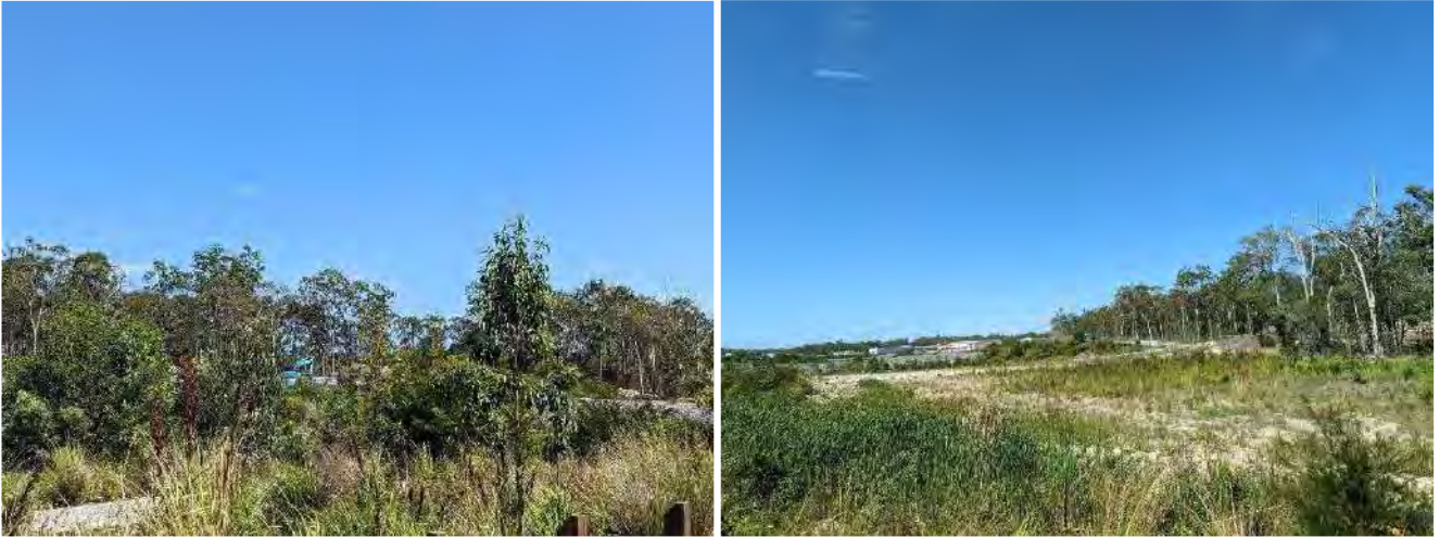
Photo Set 1: Construction and continued planting of northern Stage 1 basin and rehabilitation of waterway.
