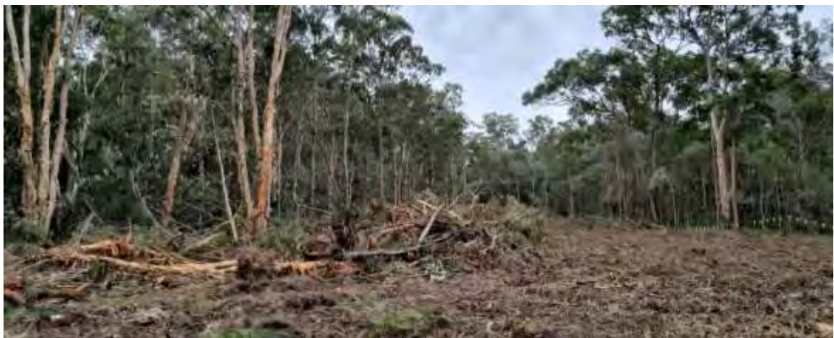
FIGURE 3- SITE DURING CLEARING
