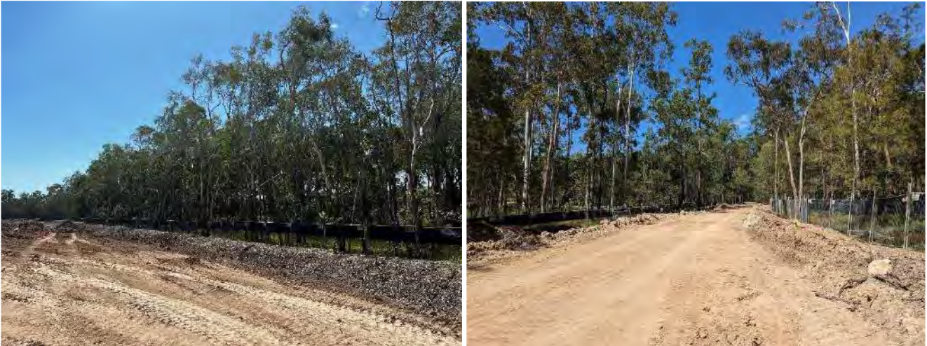
Photo Set 2: Tree protection fencing installed on construction area boundaries.
