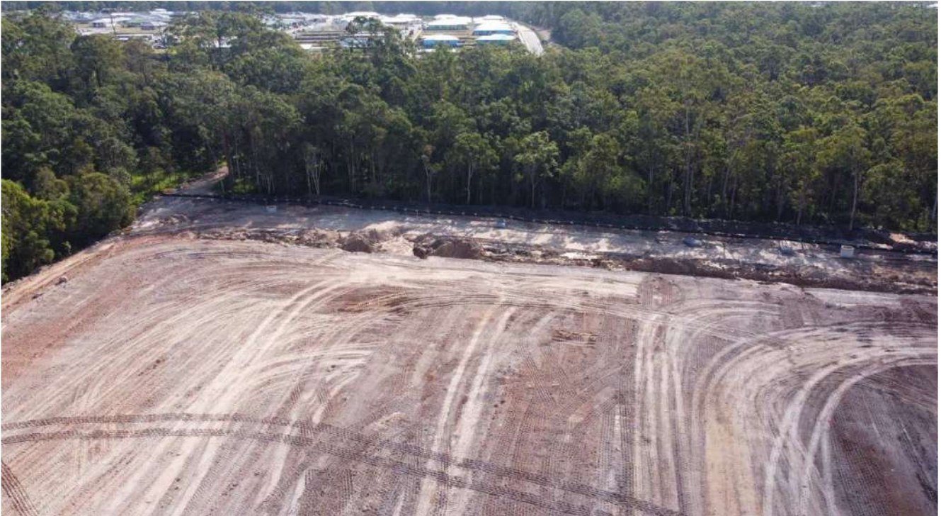
Photo 2: Temporary koala exclusion fencing installed along western boundary (4 April 2022).
