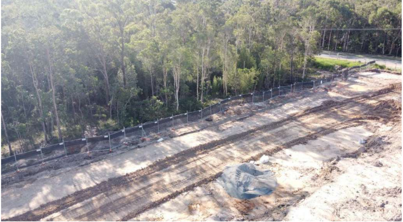
Photo 1: Temporary koala exclusion fencing installed within north-western corner (4 April 2022).
