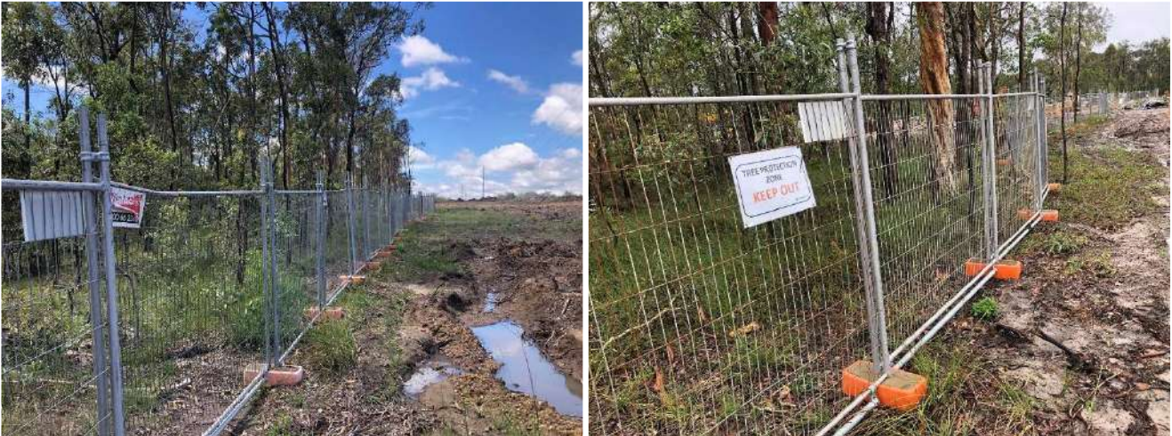
Photo Set 3: Tree protection fencing installed on construction area boundaries.
