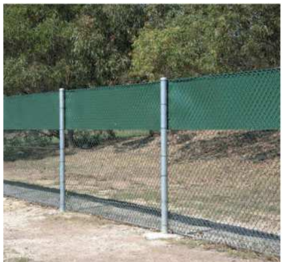
Chain wire with 600mm exclusion element
